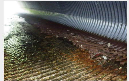
Failing Invert
