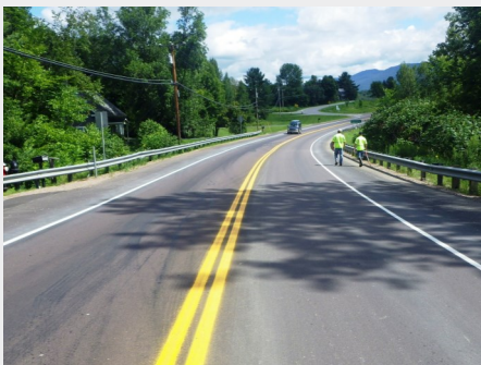
Looking North Over Bridge
